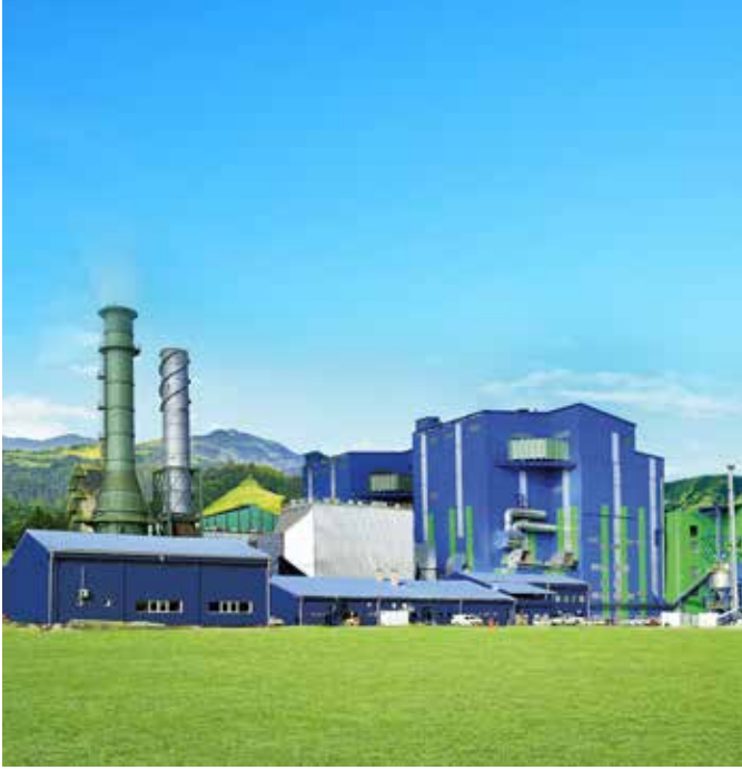
Bolu Göynük Thermal Power Plant
